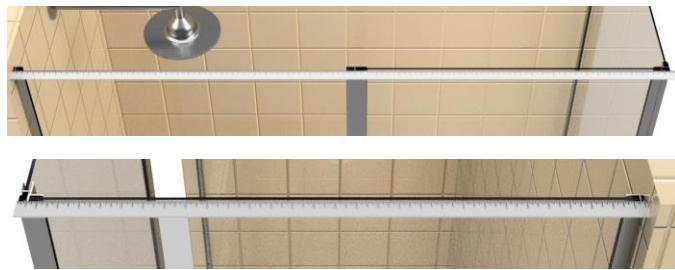
**Step 14:** Assemble headers together using supplied corner bracket and screws. Slide header assembly over wall jambs and inline post (and corner post, if applicable). Drill holes at header assembly through wall jambs and inline post. Secure with #6 x 5/8" screws.
